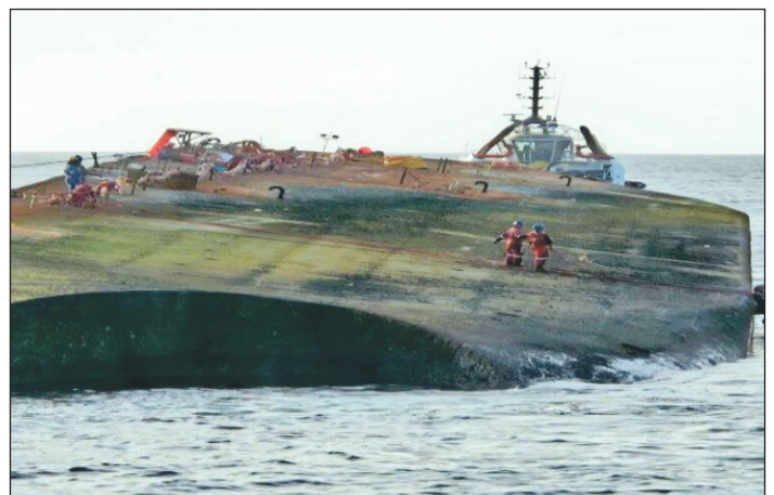
Figure 12. Workers from T&T Salvage Inc secure the overturned Gulfstream barge to tugs during the refloating exercise at Cove, Tobago in August 2024
